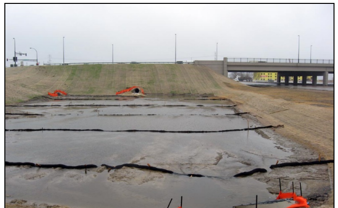
Basins are designed to filter or infiltrate stormwater
