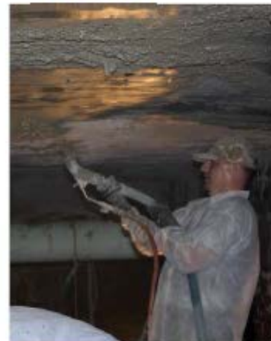
Hand sprayed application
