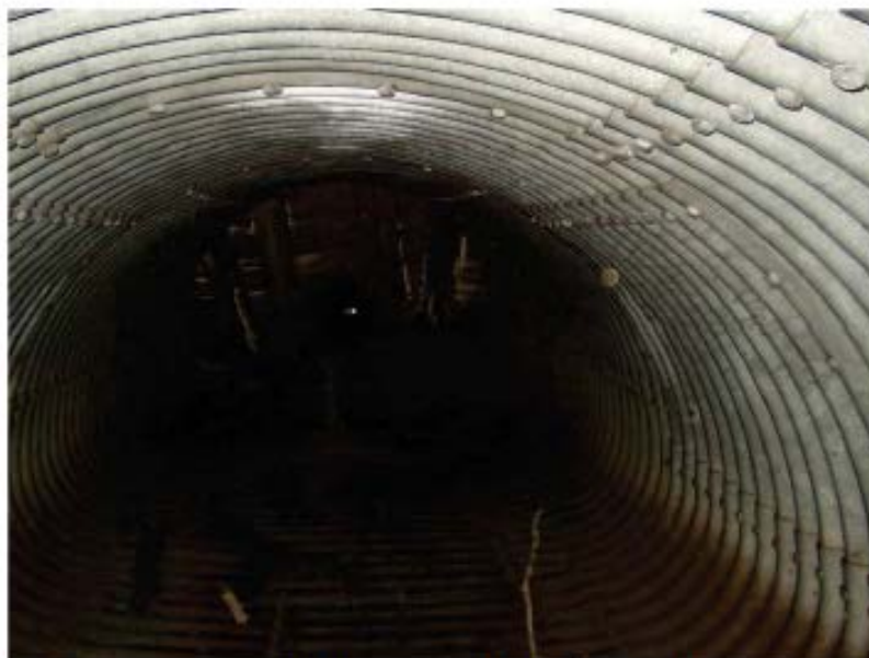
Galvanized steel plates are bolted together, was used in larger diameter culverts
