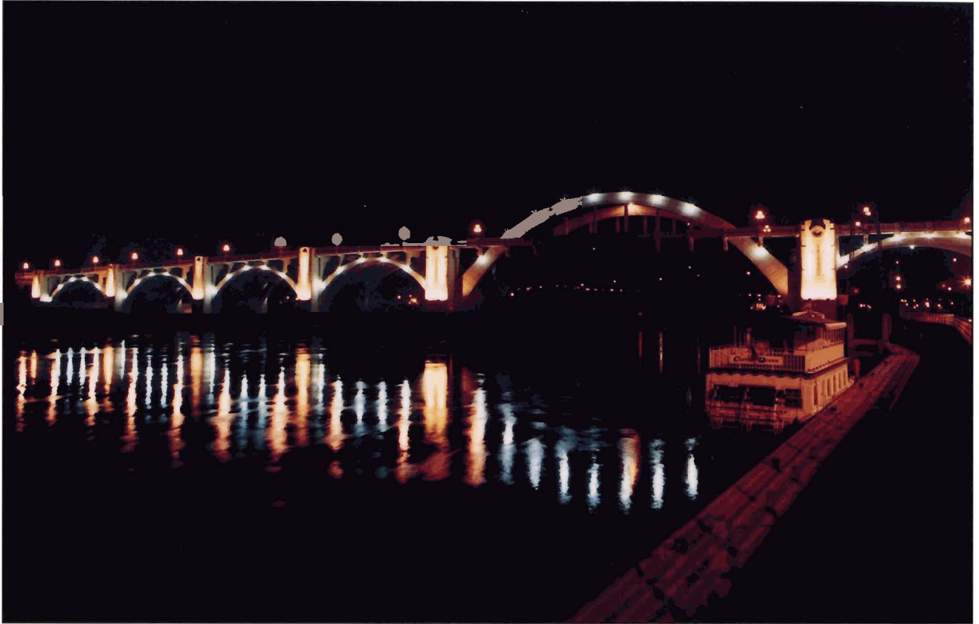
Fig. 5-1. Robert St. Bridge, St. Paul, Minnesota
