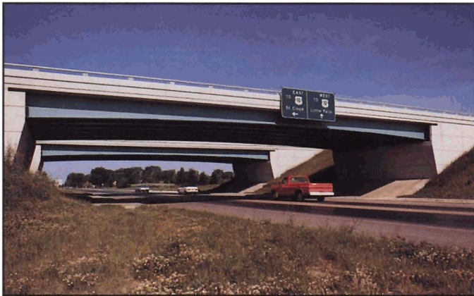
Fig. 4-16. Haunched beam contrasts with straight rail, resting on visually prominent abutments, Hwy. 10, Little Falls, Minnesota
