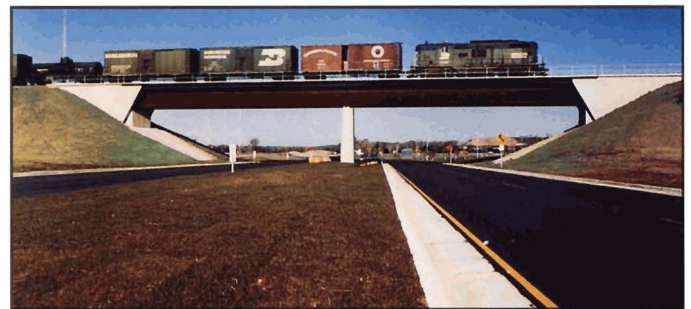
Fig. 4-13. Prominence of abutments and superstructure focuses visual attention of entire composition, Burlington Northern over Beam Avenue, Maplewood, Minnesota
