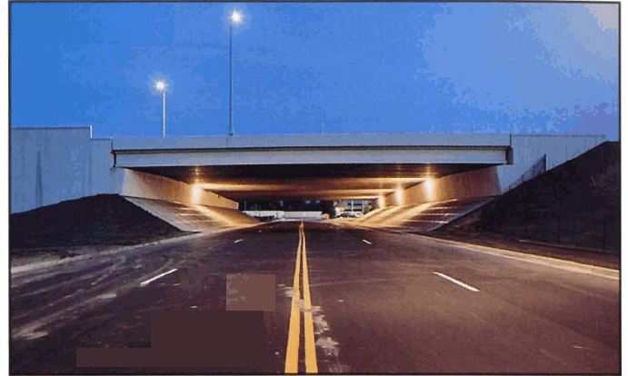
Fig. 5-32. Battered abutment face without mask wall, General Mills Boulevard over I-394, Minneapolis, Minnesota
