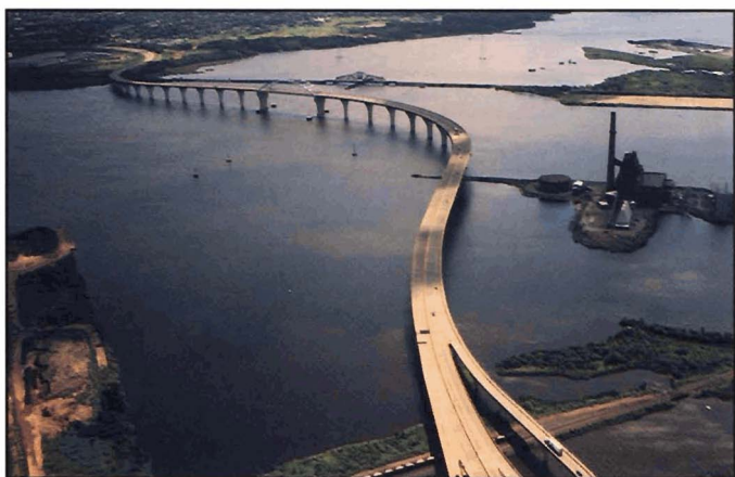
Fig. 7-7. Length and prominence of interstate bridge creates regional landmark, Bong Bridge, Duluth, Minnesota
