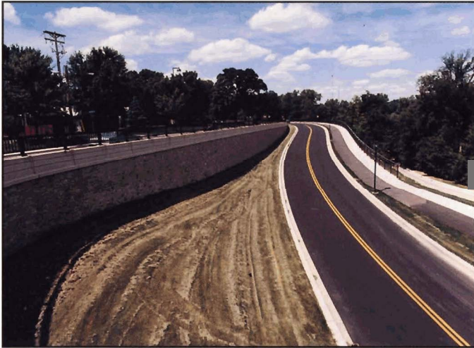
Fig. 6-19. Distance between wall and roadway is maximized to increase drivers' comfort and reduce wall height, making termination of wall logical and gradual
