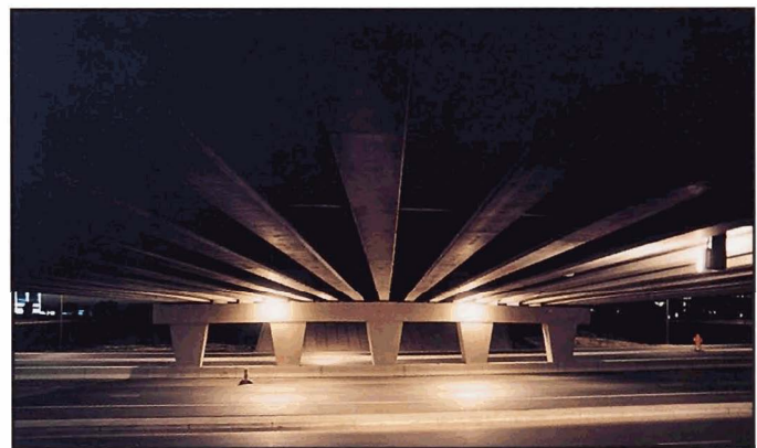
Fig. 6-17. Lighting provided beneath structure increases drivers' comfort level
