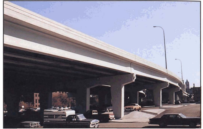
Fig. 4-4. Prestressed concrete beams used on slightly curved alignment, I-94 entrance ramp, Minneapolis, Minnesota
