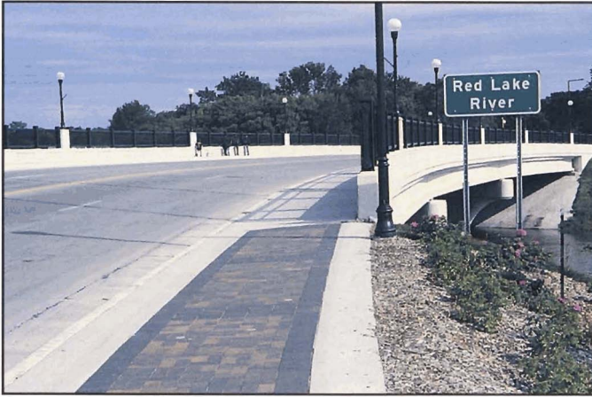
Fig. 6-28. Brick pavers used for walkway paving, Robert St. Bridge, Crookston, Minnesota
