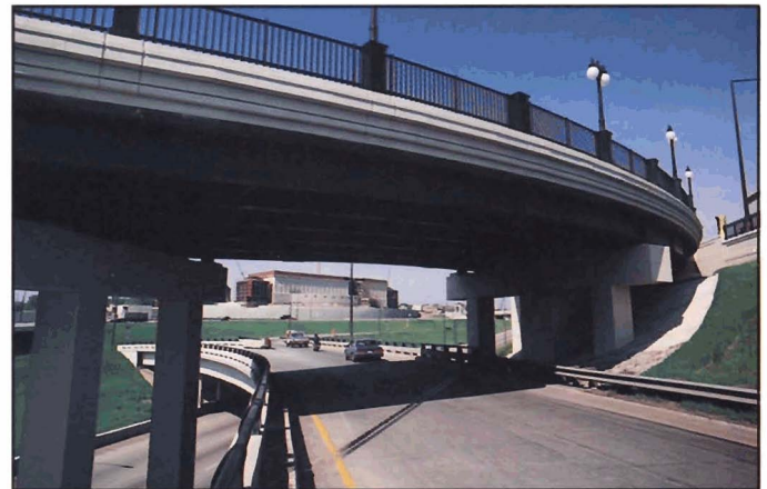
Fig. 4-5. Steel girders reflect lines of horizontally curved alignment, Minnesota
