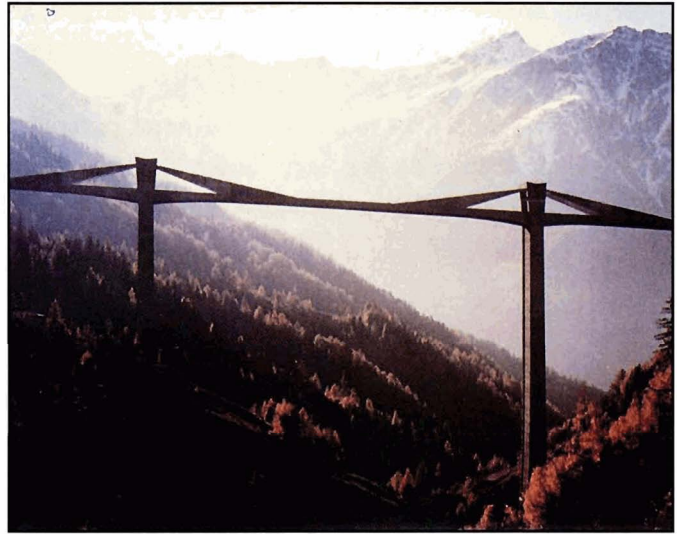
Fig. 2-13. The Ganter Bridge designed by Menn in 1980, Switzerland
