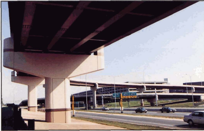
Fig. 5-6. Family of piers that vary by height, Kilebrew Drive, Bloomington, Minnesota
