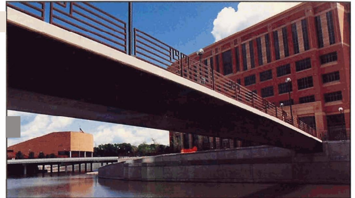
Fig. 4-22. Steel box girder provides graceful, slender presentation, Rochester, Minnesota
