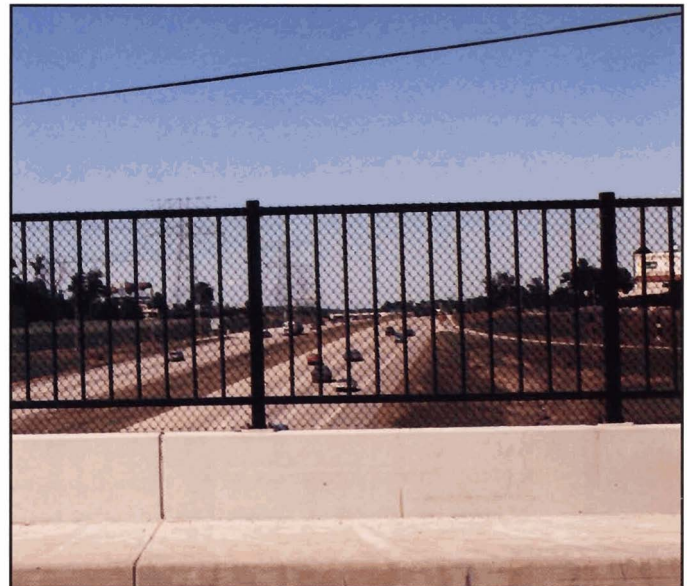
Fig. 6-11. Black screen with black frame provides consistent visual statement that is subordinate to mass and color of parapet
