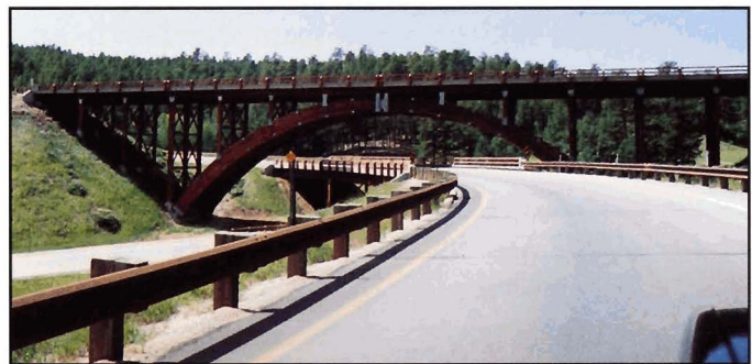
Fig. 3-6. Natural beauty of site reflected in bridge type and materials, Black Hills National Forest, South Dakota
