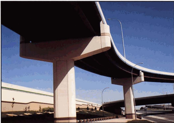
Fig. 3-4. Retaining walls and bridge elements share common visual design elements, T.H. 77 interchange, Bloomington, Minnesota
