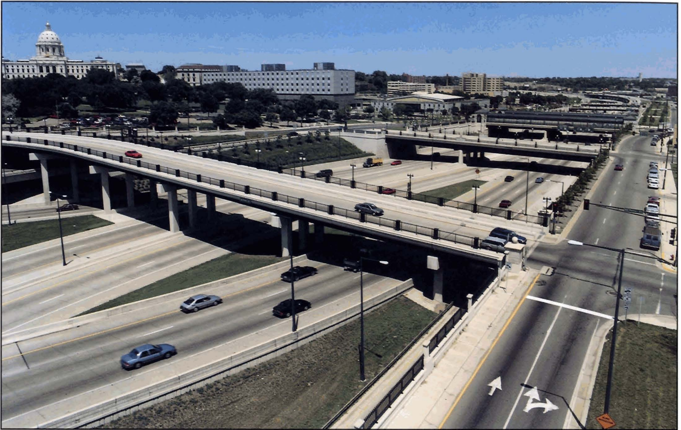
Fig. 1-1. Bridges within capital approach area, St. Paul, Minnesota
