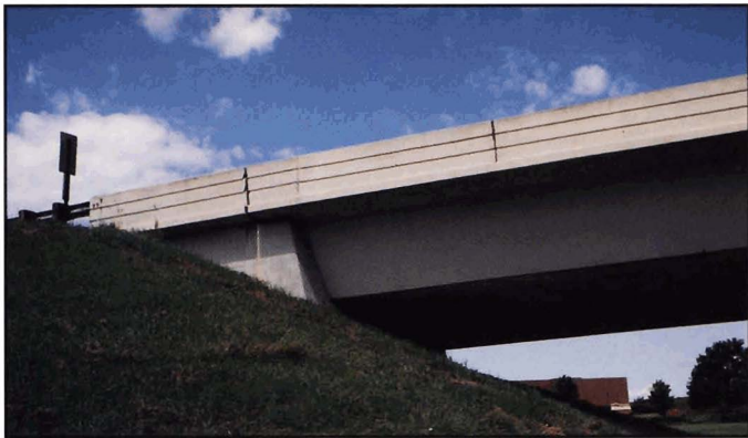
Fig. 5-34. Abutment face battered outward
