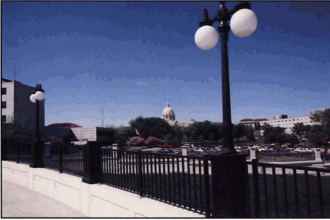
Fig. 6-10. Parapet with ornamental railing and complementary lighting produces pronounced character, St. Paul, Minnesota
