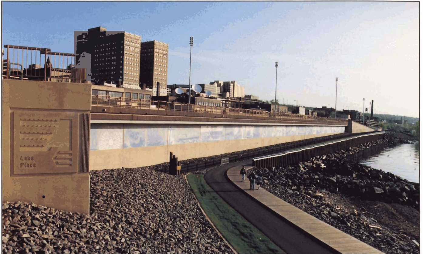
Fig. 6-1. Lake Place walkway, Duluth, Minnesota
