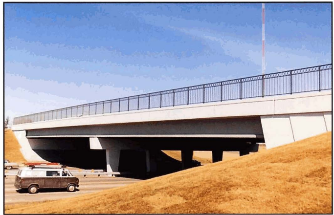
Fig. 4-15. Deck overhang creates strong shadow on fascia beam, fascia beam colored darker than abutments and rail, Victoria over I-694, Shoreview, Minnesota
