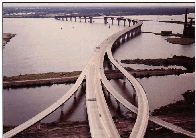
Fig. 5-5. Family of piers that vary by height, Bong Bridge, Duluth, Minnesota
