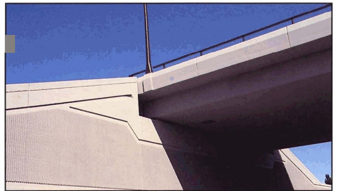
Fig. 5-47. Deep abutment, Duluth, Minnesota
