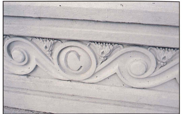
Fig. 6-25. Formliner used to create detailed sculpture in bridge parapet, Crookston, Minnesota
