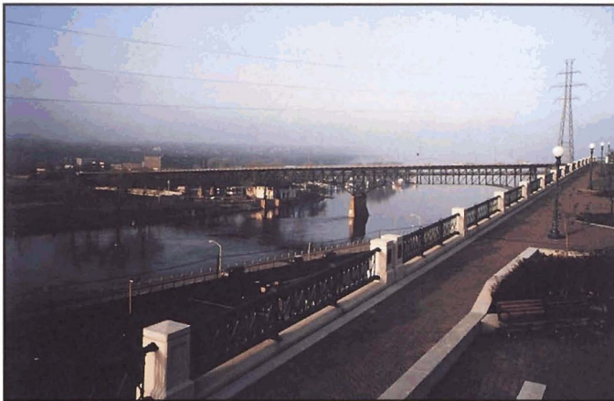
Fig. 3-10. Original photographic image of existing bridge, Wabasha St. Bridge, St. Paul, Minnesota
