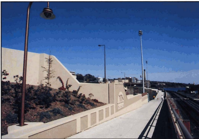
Fig. 6-24. Recess rib rustication and host city icon provide pedestrians and drivers with visual interest, Duluth, Minnesota
