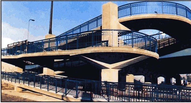
Fig. 6-7. Fine detail and color of pedestrian railing add to what otherwise might be a mundane ramp, Hennepin Ave. Bridge, Minneapolis, Minnesota
