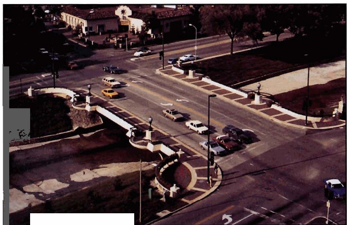
Fig. 2-16. Wornall Road Bridge – sensitive to urban setting, Missouri
