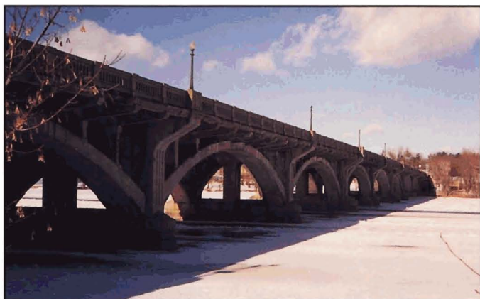
Fig. 7-8. Photograph of bridge after its initial construction, Anoka/Champlin Bridge, Minnesota
