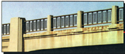
decorative metal railings
