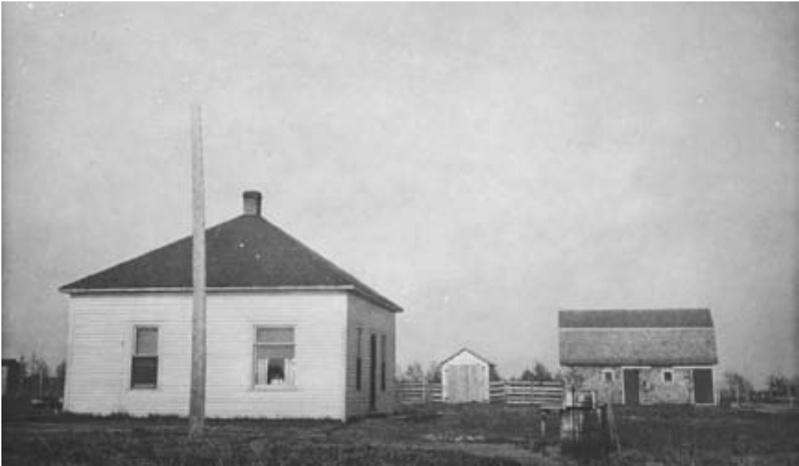
Farms in Area 8 – northeastern Minnesota’s cutover region – averaged 103 acres in 1939, considerably smaller than the state average of 165 acres. Most farm buildings were modest as well. Near Graceton, Lake of the Woods County, circa 1919. (MHS photo)
