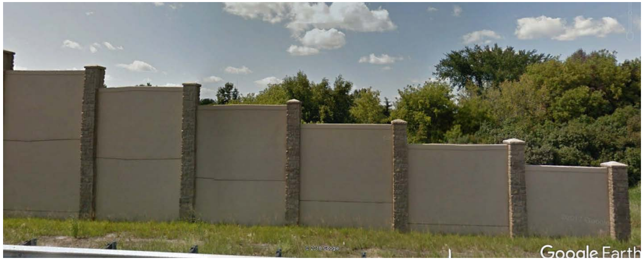
Figure 1: Tapering of a concrete noise wall located in Eagan, MN.
