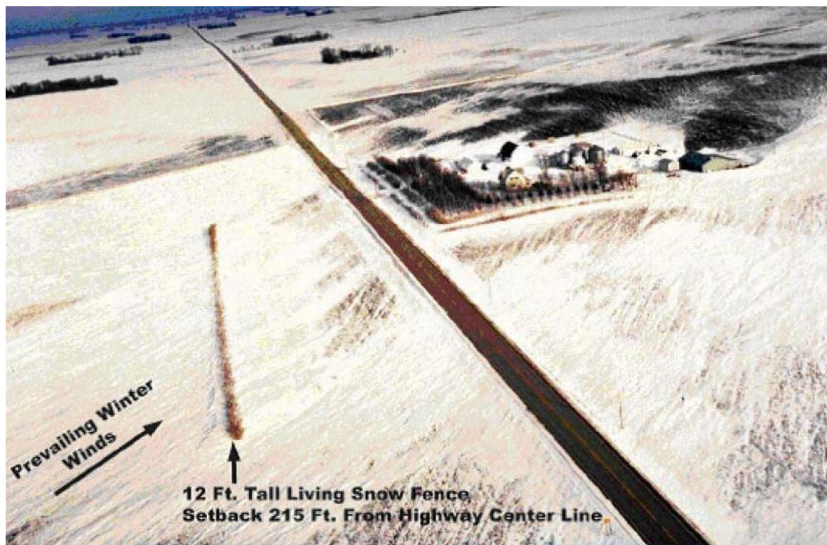
FIGURE 9: LIVING SNOW FENCE
