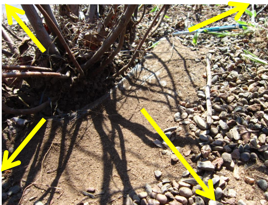
FIGURE 12: X-SHAPED SLIT IN GEOFABRIC FOR WEED BARRIER
