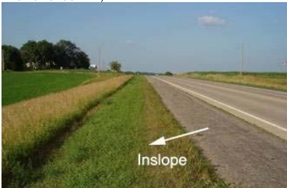
FIGURE 5: INSLOPE (TYPICALLY BEGINS 2-4 FEET FROM EDGE OF SHOULDER)
