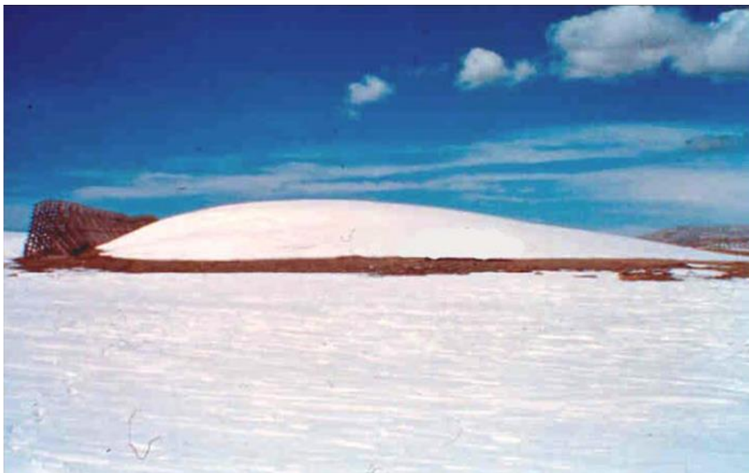
FIGURE 14: STRUCTURAL SNOW FENCES (PHOTO COURTESY OF DR. RON TABLER OF TABLER & ASSOCIATES)
