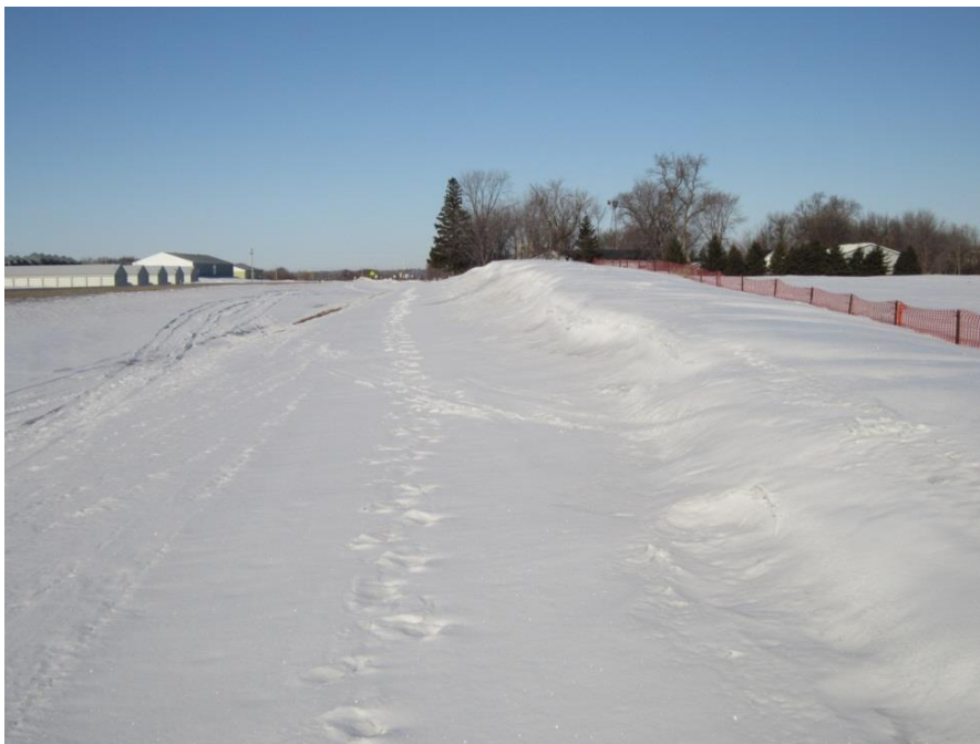
FIGURE 17: A FOUR FOOT TALL PLASTIC ORANGE SNOW FENCE USED TO REDUCE BLOWING AND DRIFTING SNOW ON THE HIGHWAY
