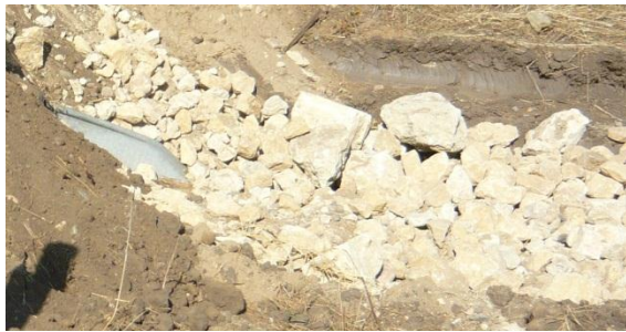
FIGURE 3: RIPRAP DETAILS
