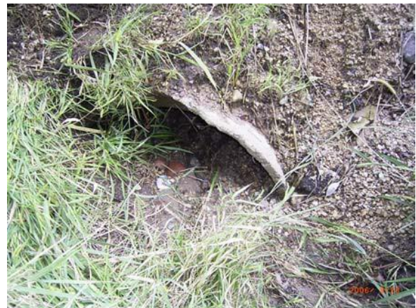
FIGURE 2: SILT/DIRT-FILLED CULVERT
