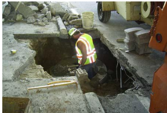
FIGURE 11: MANHOLE REPAIR OPERATION
