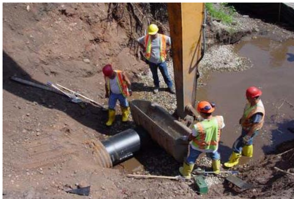
FIGURE 9: TYPICAL SLIP-LINING OPERATION TO REPAIR A CULVERT
