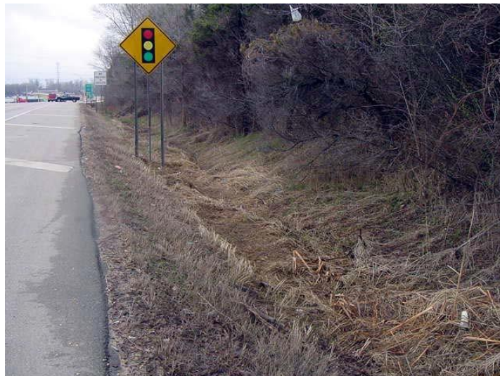
FIGURE 15: TYPICAL ROADSIDE DRAINAGE DITCH
