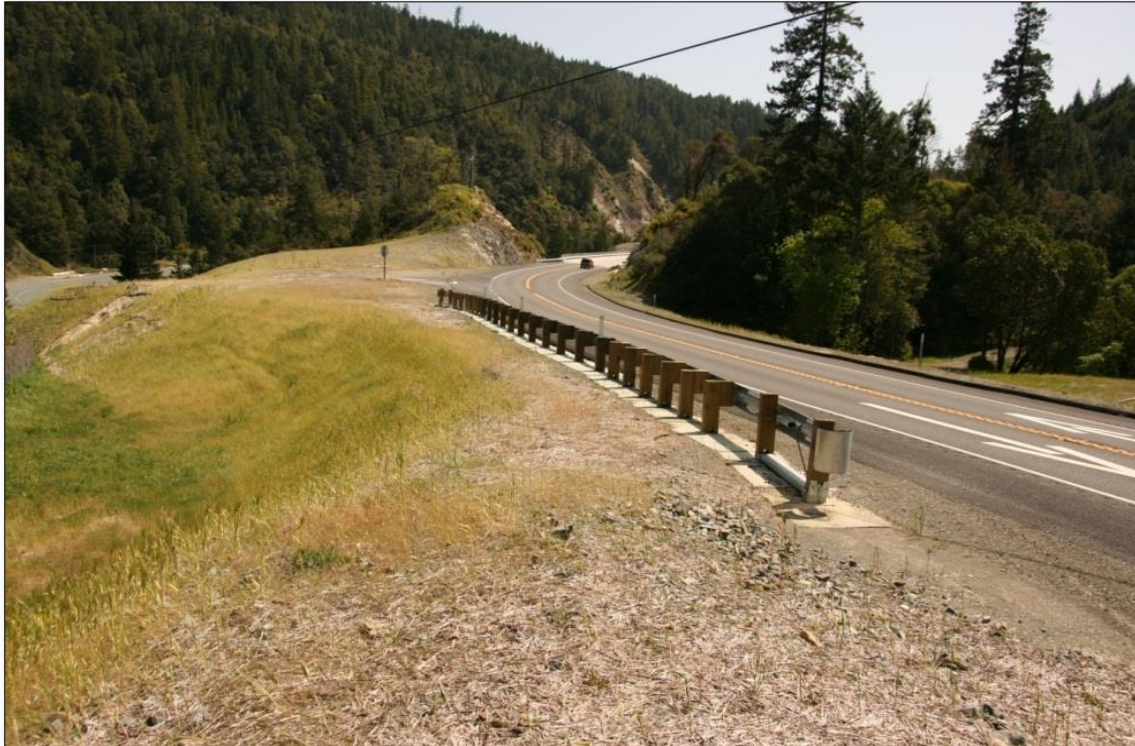
Figure 2-8: Final Condition, Confusion Hill TDA Fill Volume
