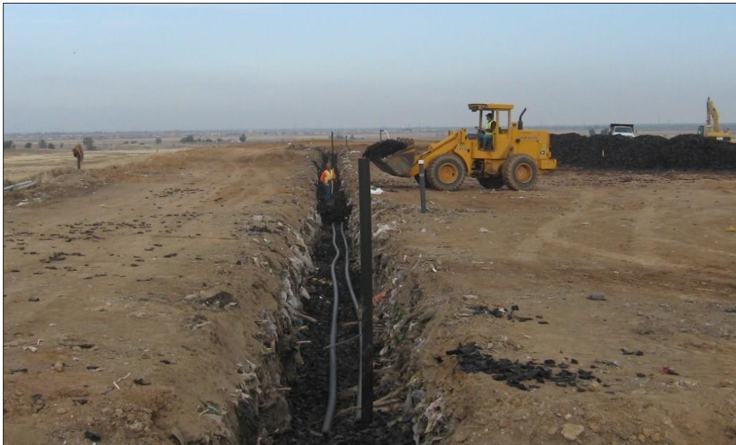
Figure 2-30: Kiefer Landfill TDA and Piping Placement
