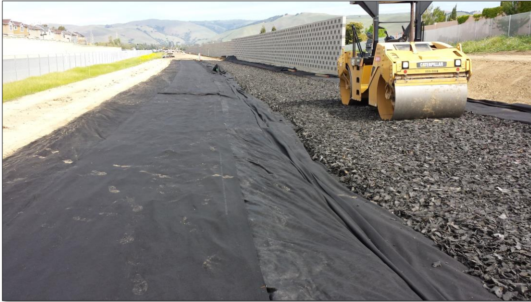
Figure 2-26: BART TDA Placement
