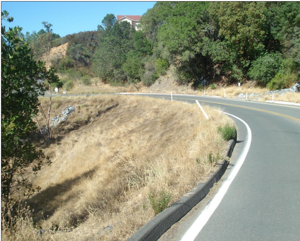
Figure 2-16: Completed Marina Drive Slide Repair TDA Project
