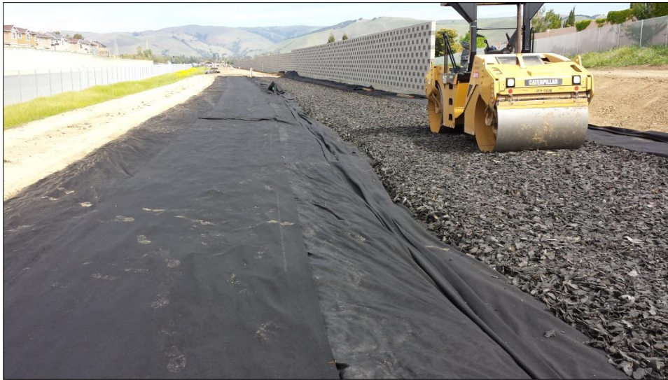
Figure 4-3: Drum Roller at the BART Warm Springs Rail Extension Project
