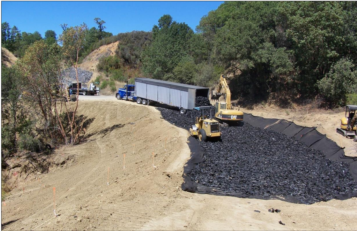
Figure 2-14: TDA Delivered, Spread, and Compacted on Marina Drive
