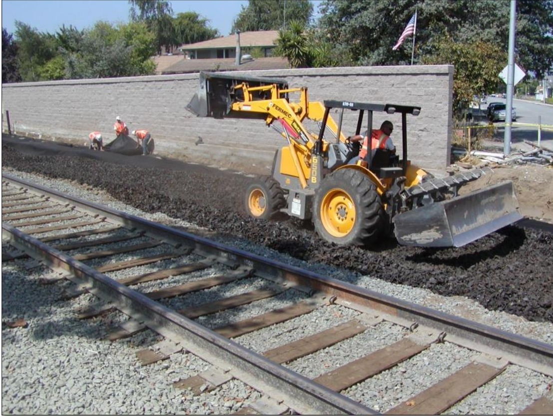
Figure 2-25: Spreading Type A TDA During Construction
