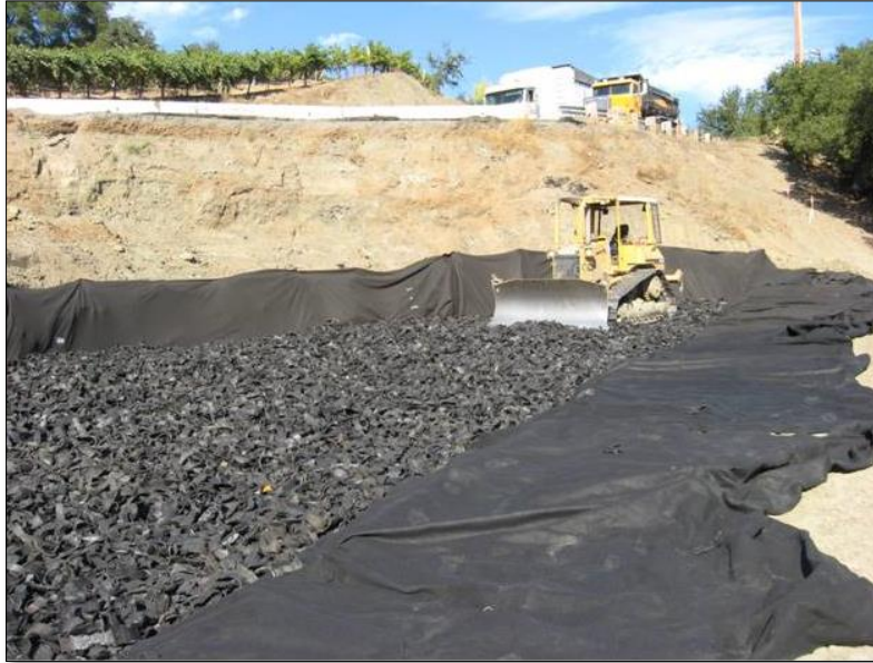
Figure 2-22: Spreading TDA Above Geotextile in Sonoma County
