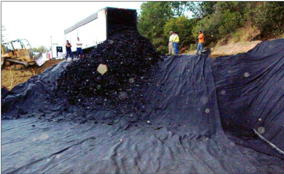
Figure 2-13: Walking Floor Semi-Truck Unloading TDA onto Geotextile
