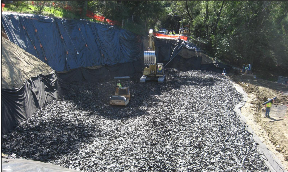
Figure 2-18: TDA Placement and Compaction at Sonoma Mountain Road
