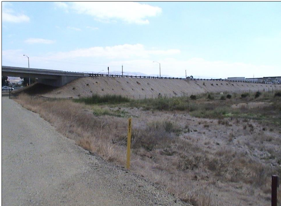
Figure 2-4: Final Dixon Landing TDA Embankment
