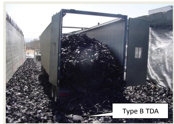
Figure 1-1: Type B TDA Used as Retaining Wall Backfill Material
