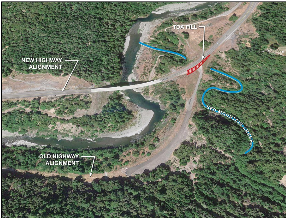
Figure 2-5: Confusion Hill Backfill Project Overview
