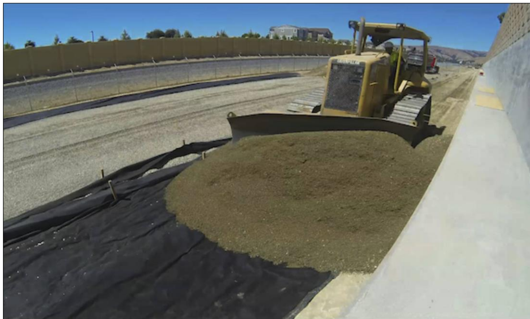
Figure 2-27: BART Sub-Base Over TDA Placement
