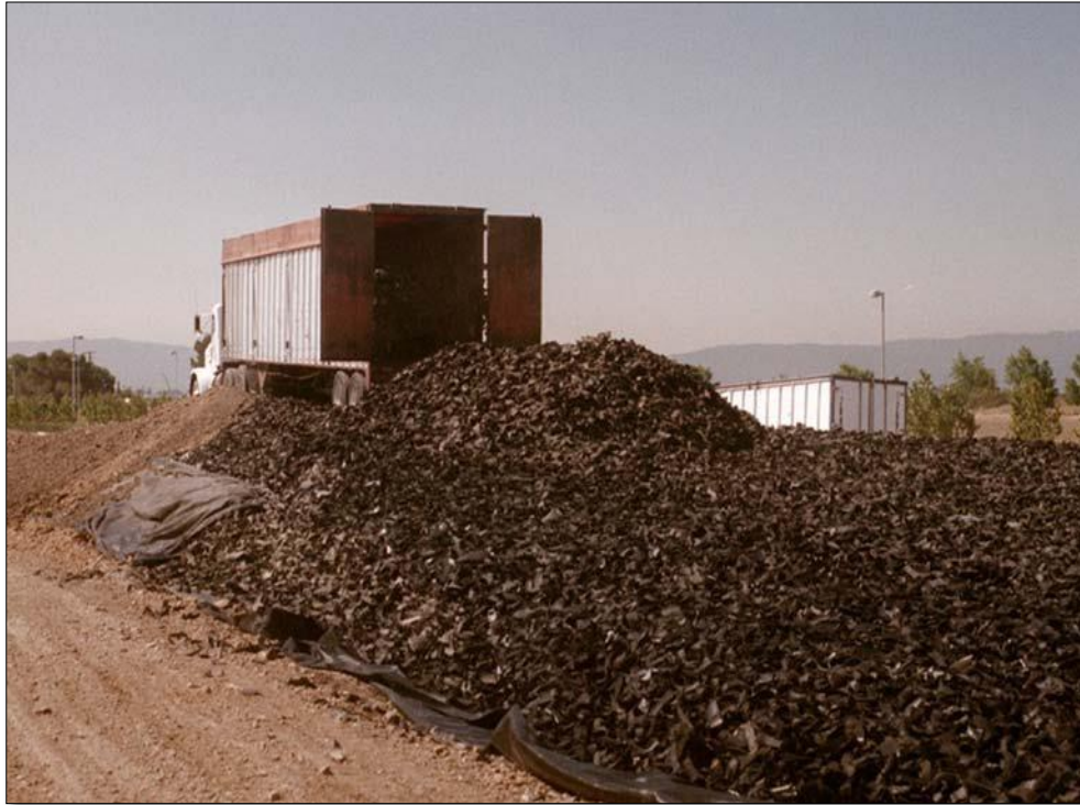
Figure 2-1: Unloading TDA from Walking Floor Trailer
