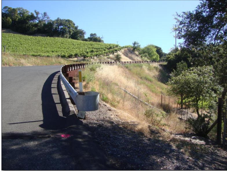
Figure 2-23: Completed Geysers Road Slide Repair
