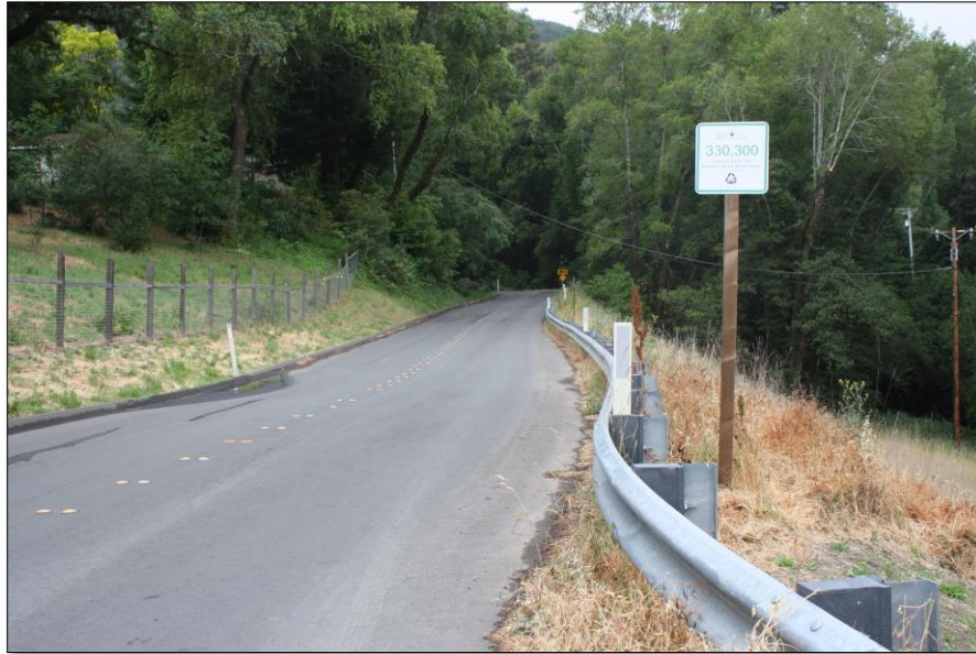
Figure 2-20: Final Sonoma Mountain Road TDA Slope Repair Project
