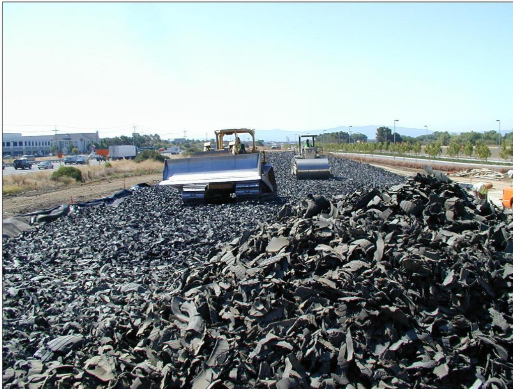
Figure 2-2: TDA Being Compacted at Dixon Landing
