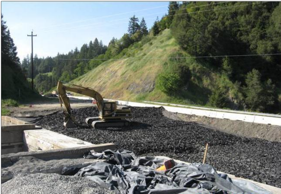
Figure 2-7: TDA Placement at Confusion Hill Site
