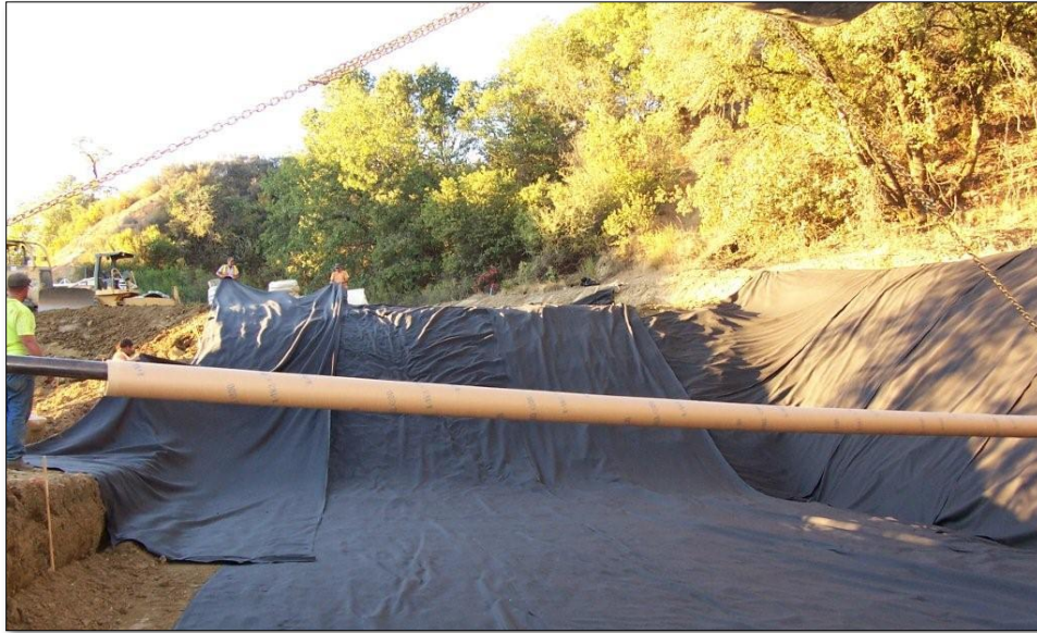
Figure 2-12: Placement of Geotextile During a TDA Slope Repair
