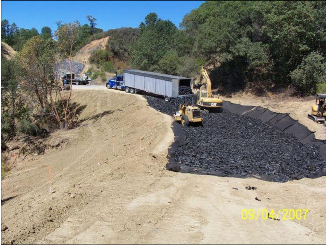
Figure 4-1: Walking Floor Trailer Unloading for Marina Project
