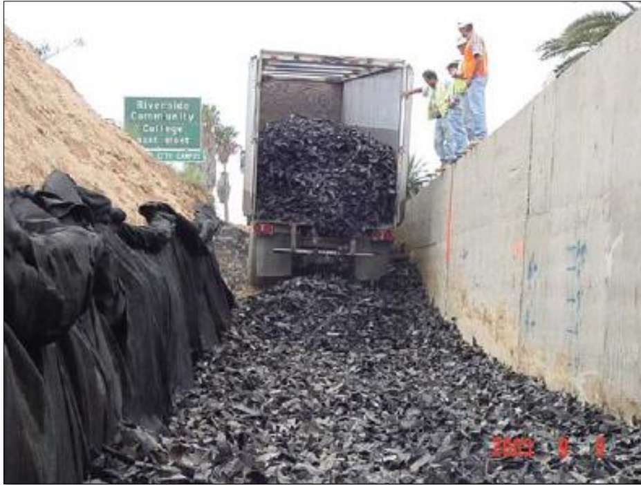
Figure 2-9: Typical TDA Delivery for Retaining Wall Backfill
