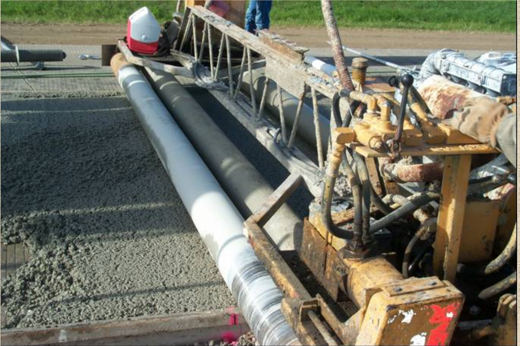
ROLLER SCREED FIXED FORM PLACEMENT
