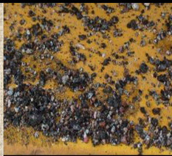
b) Agents Vacuumed from MnROAD Pervious Pavements
