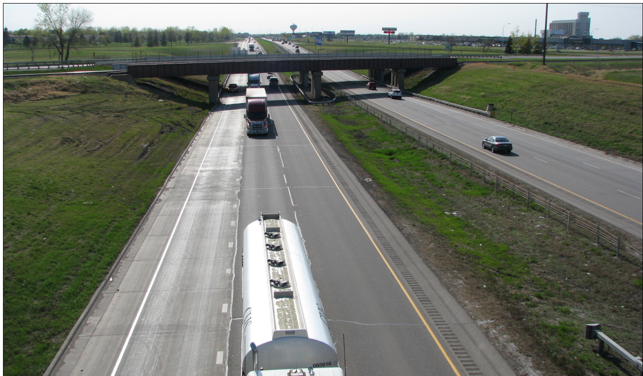
Interstate 94 is a critical connection for Pactiv and other businesses in District 4.
