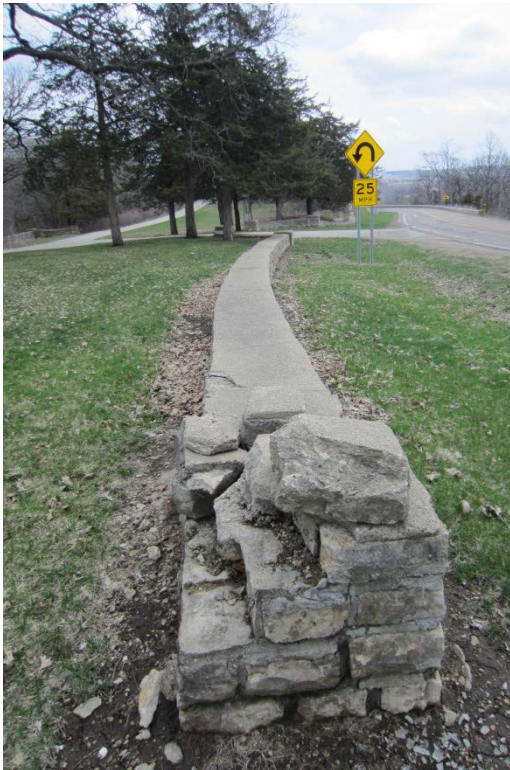
4.5 – Vehicle impact at west end of South Entrance Walls
