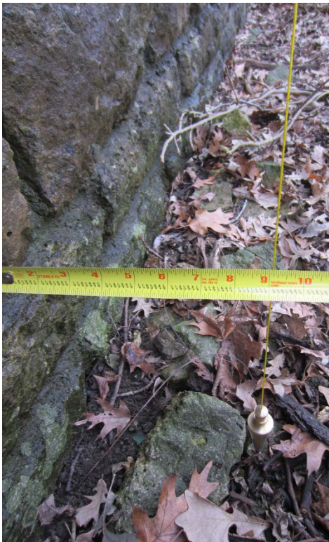
4.6 – West end of North Overlook Wall is out of plumb by 9-1/4" (above left) at the west pier is and the east pier is out of plumb by 10-3/4" (above right)
