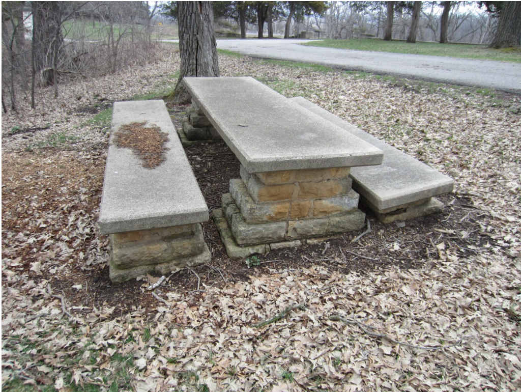
4.8 – Center Table with undermined bench
