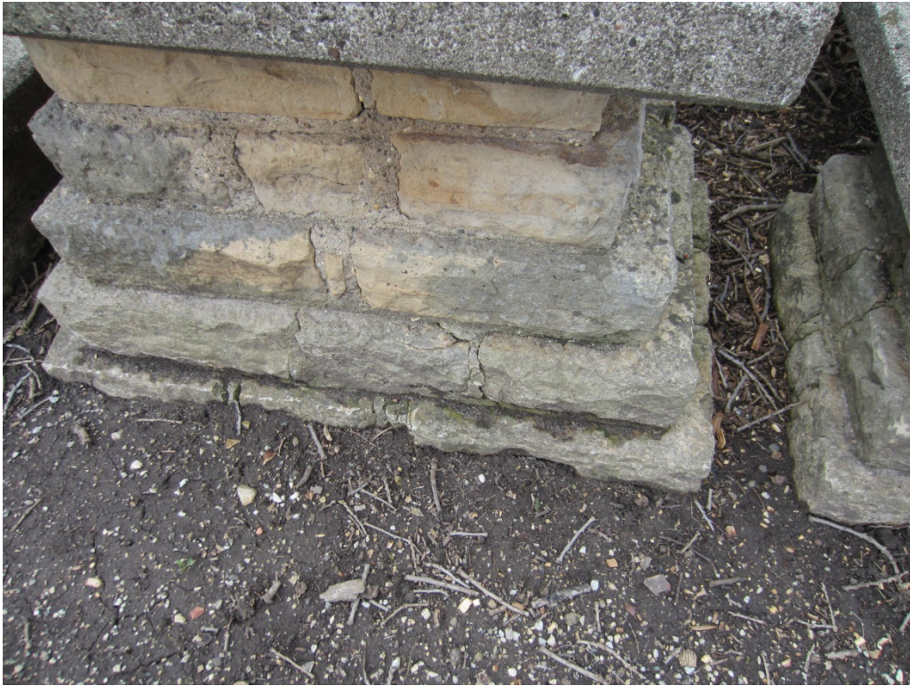
4.8 – Center Table with stone deterioration
