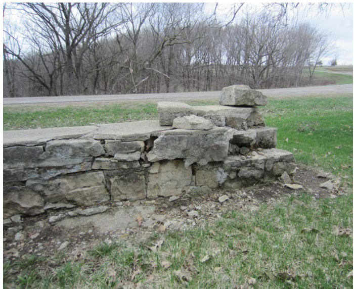
4.5 – Vehicle impact at west end of South Entrance Walls
