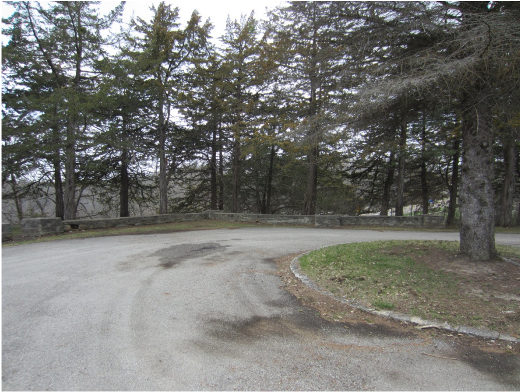
4.7 – Bituminous deterioration
