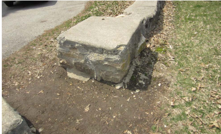
Unpaved opening through East Overlook wall
