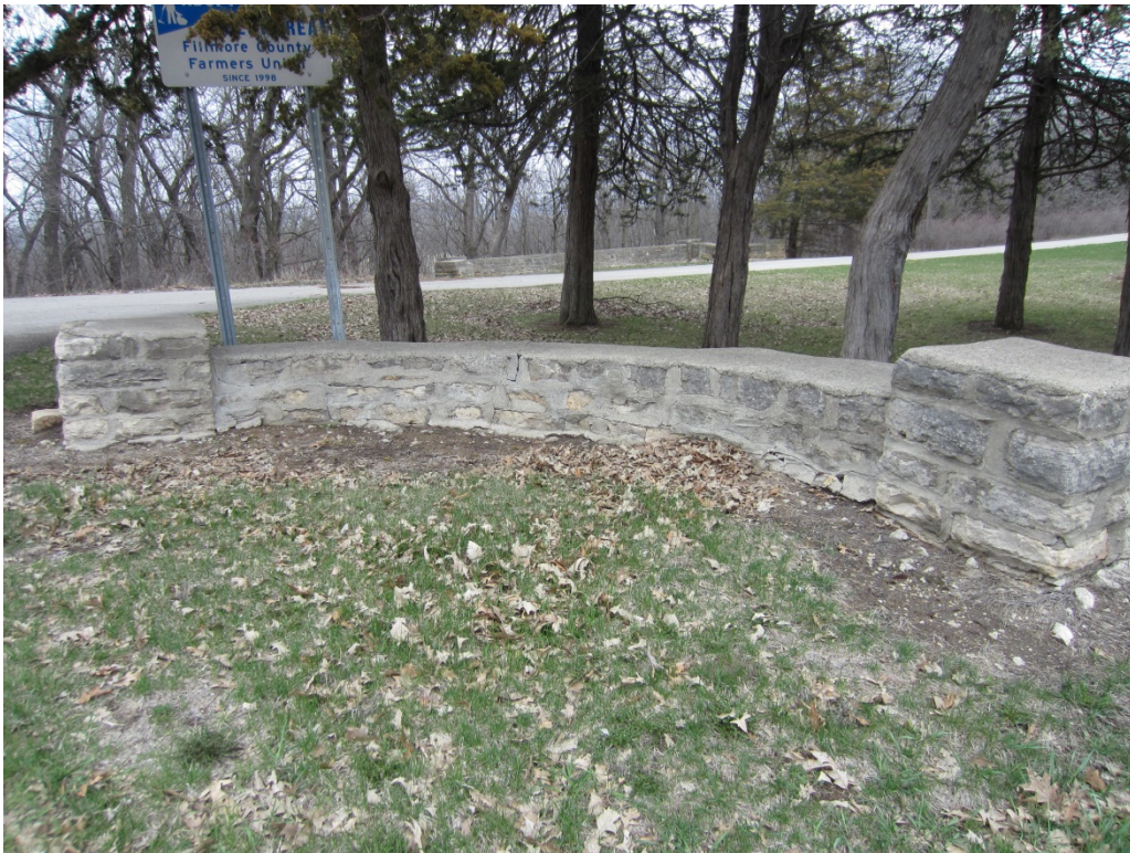
4.5 – Mortar cap and mortared joints of curved walls at Historic Entrance
